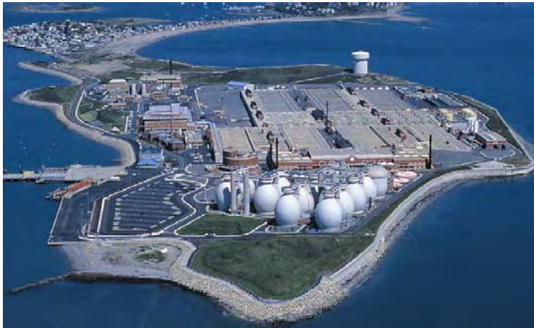
Figure FS-1: Aerial view of the Deer Island Treatment Plant
