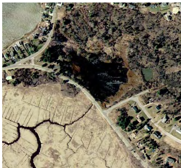
Figure 5-A: 2001 pre-restoration aerial photo of tide-restricted marsh (ponded with fresh water), Ipswich Little Neck Road
