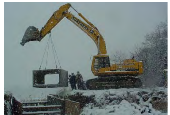
Figure FS-4: Installing the box culvert at Damde Meadows, Hingham
