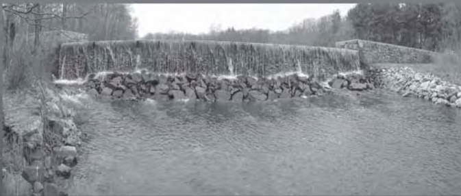
Foundry Pond Dam, Weir River, Hingham
