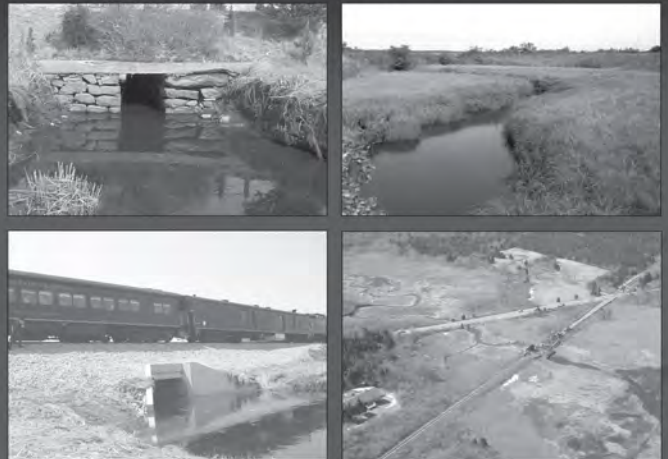
In-progress: Bridge Creek II
