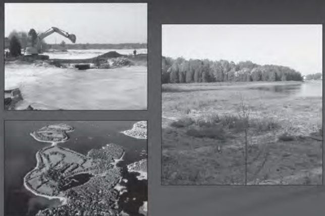
Completed project: Damde Meddowes
